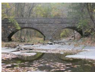
An old arch bridge
