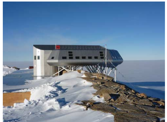
Fig. 3. View to the north of the Utsteinen Ridge and the Princess Elisabeth Station. The main wind direction is from the east (right side of the picture). Drifting snow fills the west side (left side of the picture) of the ridge. The main structure is 22 by 22 m and elevates 2–5 m above Utsteinen Ridge.
